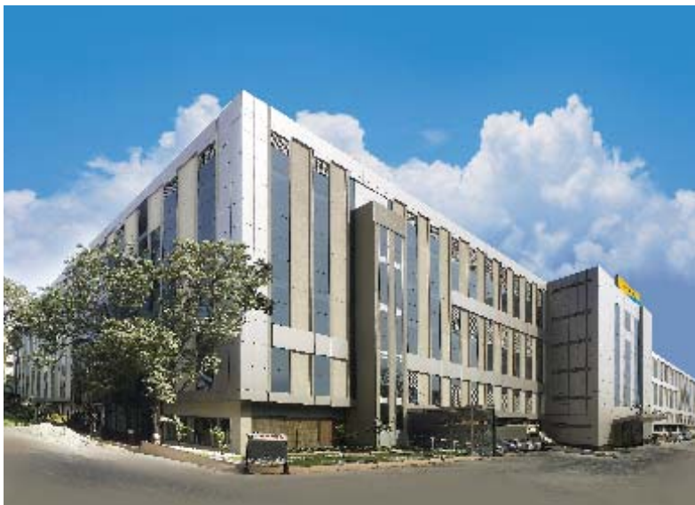
Switchgear Factory, Mumbai
